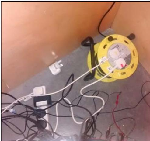
Here is an example of “daisy chaining” where one extension system (multi-way bar extension) plugged into another (cable reel) causing it to become overloaded.
